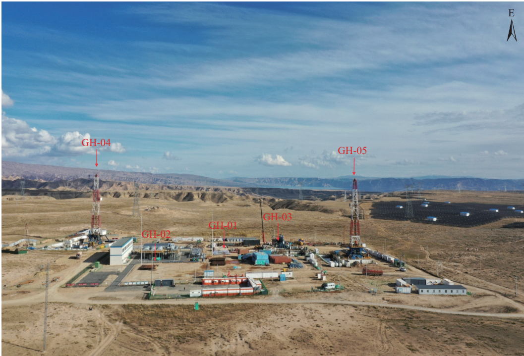
Fig. 8. HDR exploration, experimental development, and generation test site in the Gonghe Basin, Qinghai Province.
