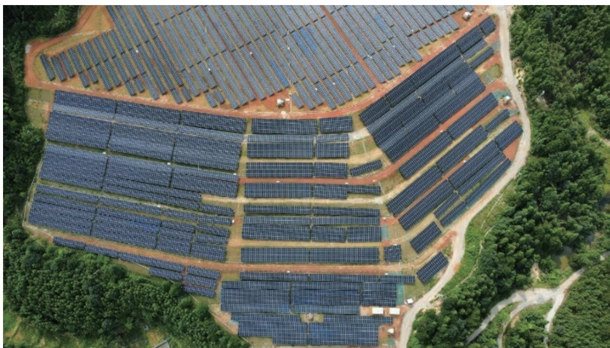
Fig. 3. Xintianling tungsten mine distributed photovoltaic project (from https://solar.in-en.com/html/solar-2457916.shtml ).
